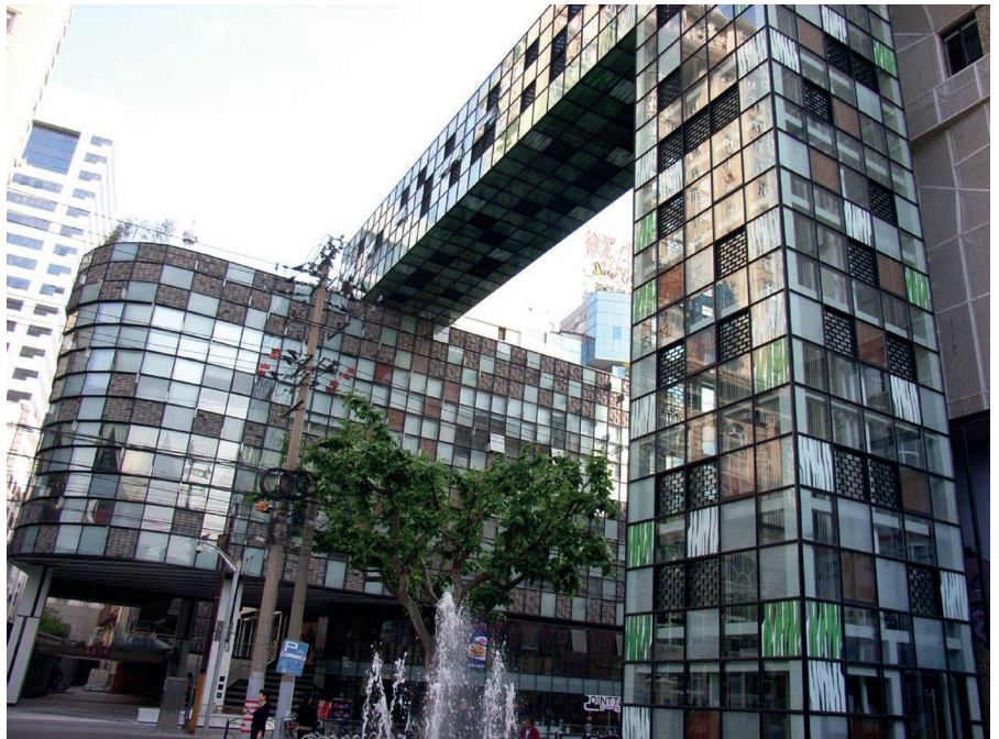
Figure 5: The "Bridge of Creativity" at Bridge 8, linking two buildings across the street
